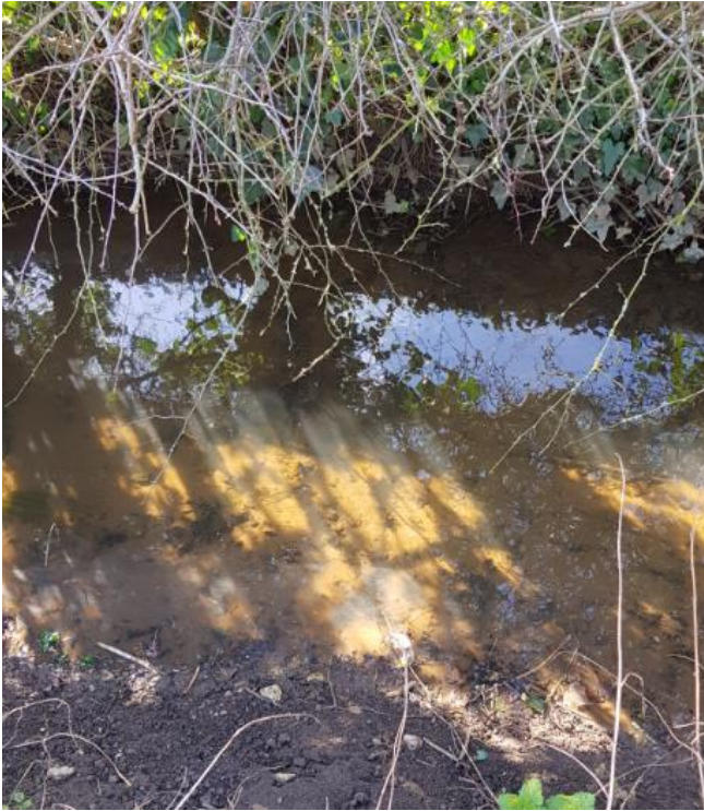
Fairstead Drove drain opposite Playing field. 24 Feb 21 Heavily silted and water depth approx. 5 inches.
